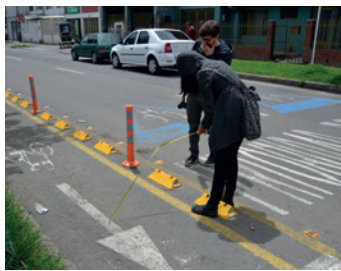
Flexible bollards in Bogota help to keep vehicles out of the bike lane
