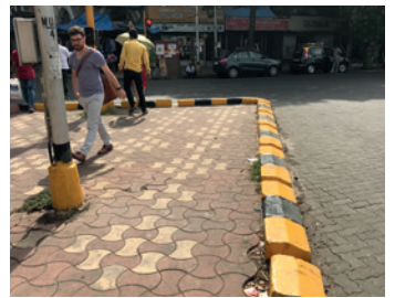
Concrete curbs provide protection for pedestrians.
