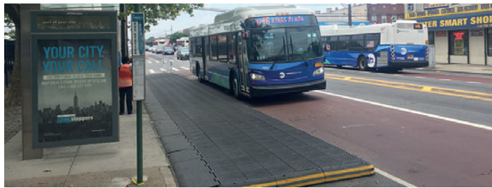
A rubber platform provides safe space for passenger boarding in New York City
